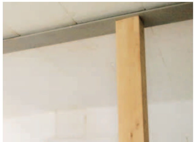
Fig. 6: A linear thermal bridge in formation. If the steel beam is not additionally integrated into the insulation, condensation is to be expected.
